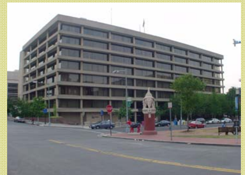
WAMATA Building Washington, DC Over 45,000 sq ft 7-mil clear with mechanical attachment system.
