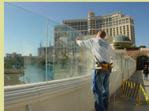
Las Vegas, NV All Las Vegas strip bridges and elevators are coated with a anti graffiti film that XInt Tint maintains.
