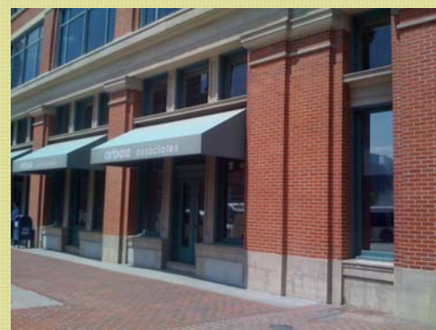
Baltimore, MD Inner Harbor office building with graffiti film. Large expensive windows that are in a high traffic area. The least expensive alternative.
