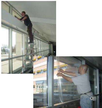
Professionally Installed And Backed
